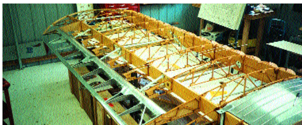
Above: Typical fabric covered wooden wing under construction.
